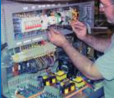
Electric Boards Assembly
